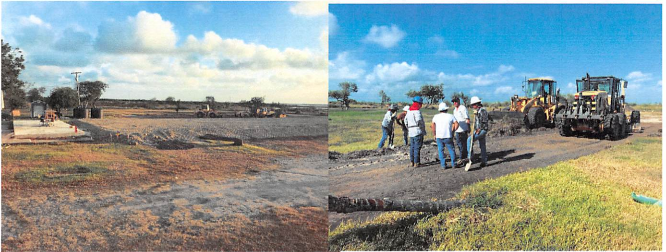
Raised pad for the slab and prepping the site.
