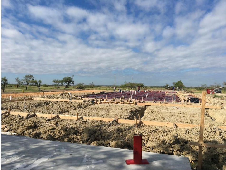
Early August 2019 – Preparing for Foundation
