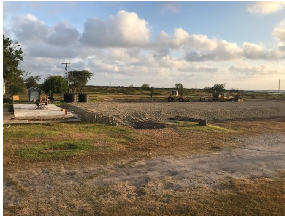
Late August 2019 – Preparing the Pad
