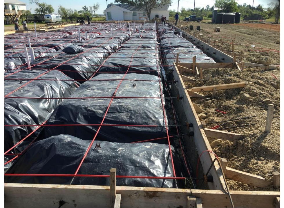
Late August 2019 – Vapor Barrier and Cables
