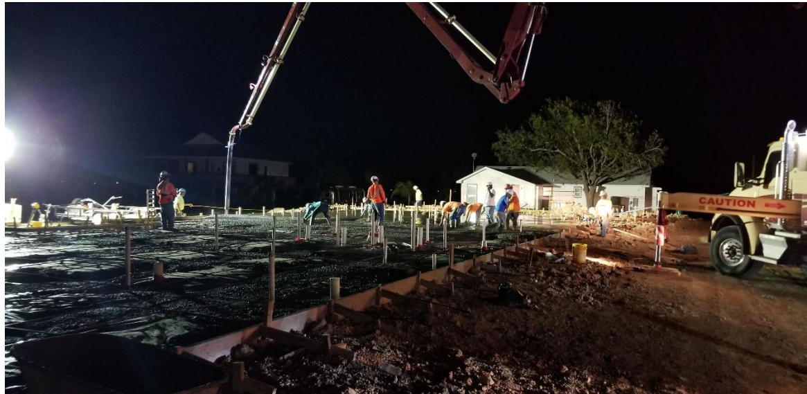
October 2019 – Pouring the Foundation!
