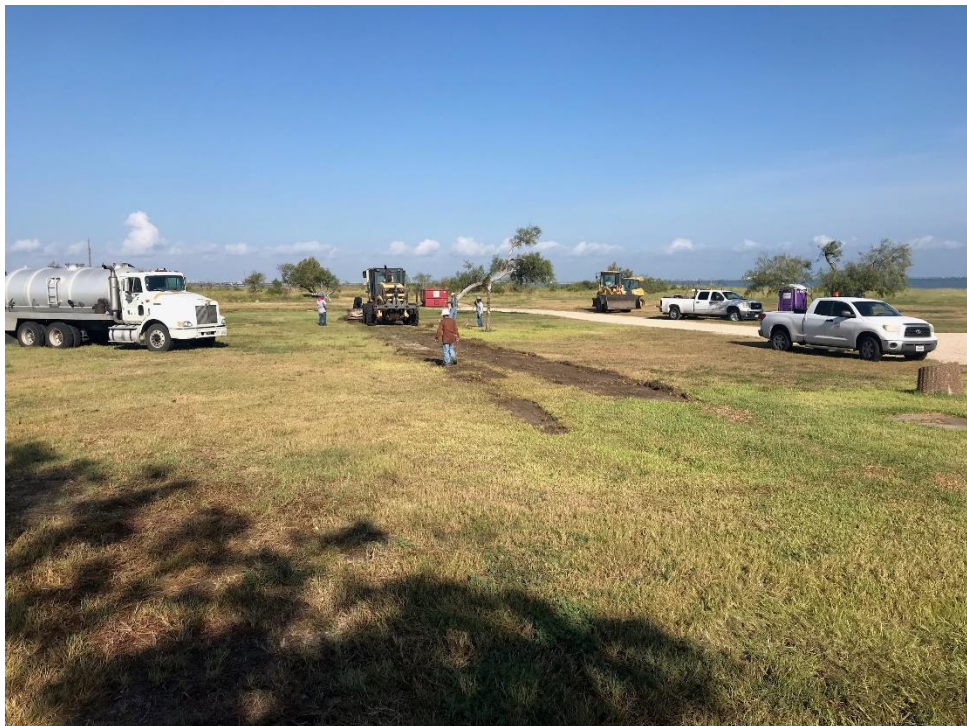
Early August 2019 – Groundbreaking
