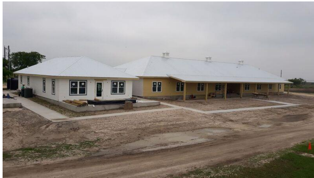
April 2020 – Painting, Walkways
