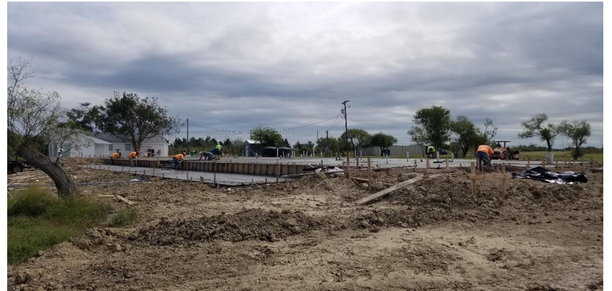
October 2019 – Rough Plumbing
